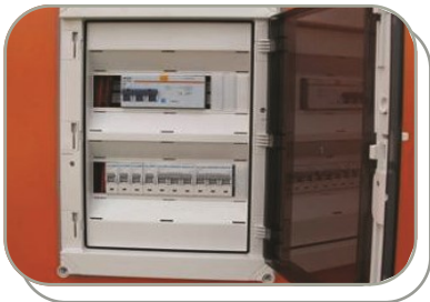
Main switch box
